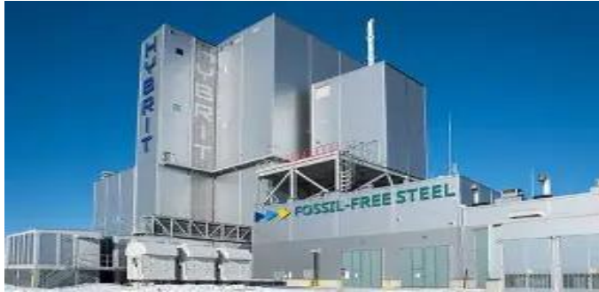
Site visits to First-of-a-kind industrial installations
